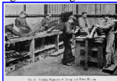
Fig. 12. Making Segments of String of First Turbine
